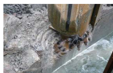
Drilling the existing RC Revetment
