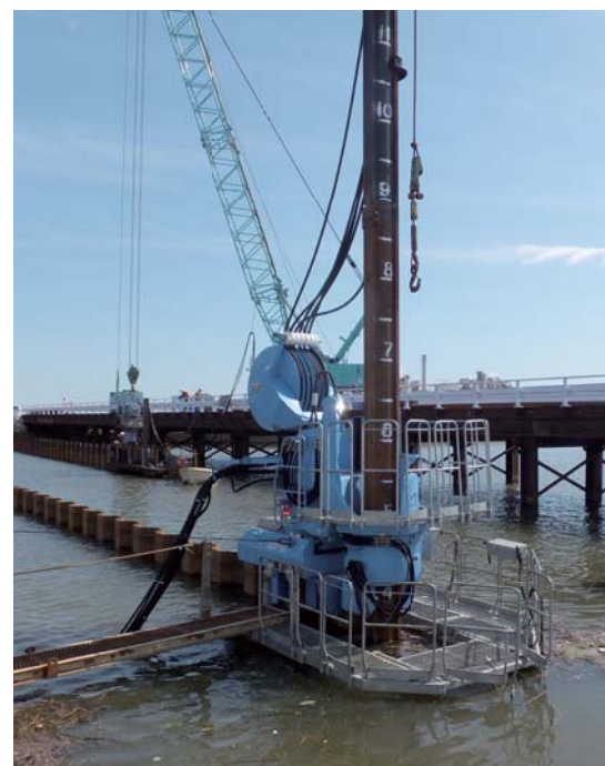
Drilling the existing RC Revetment
