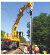
The choice of a vibrator being based on several parameters (length and type of profile, type of ground, etc. ..).
